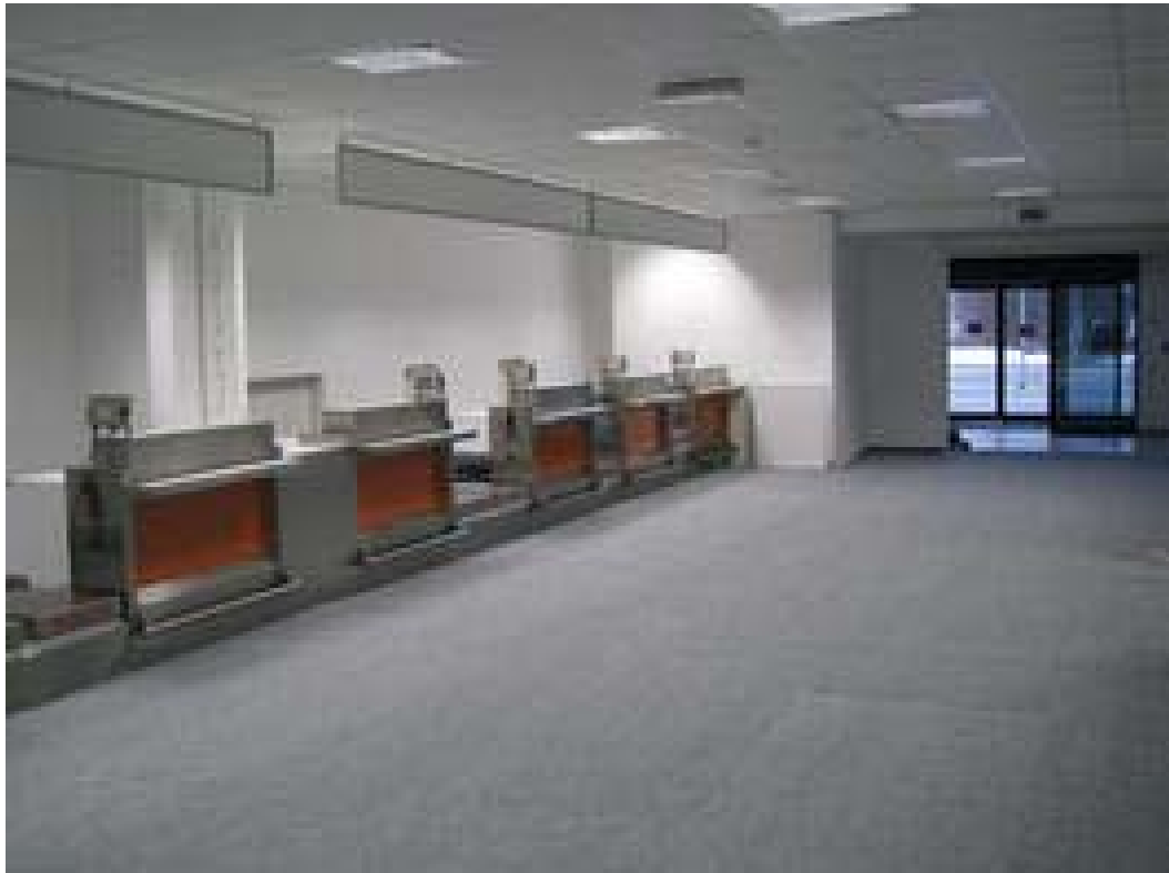
Check-In Counters (neutral, immediately after installation)
