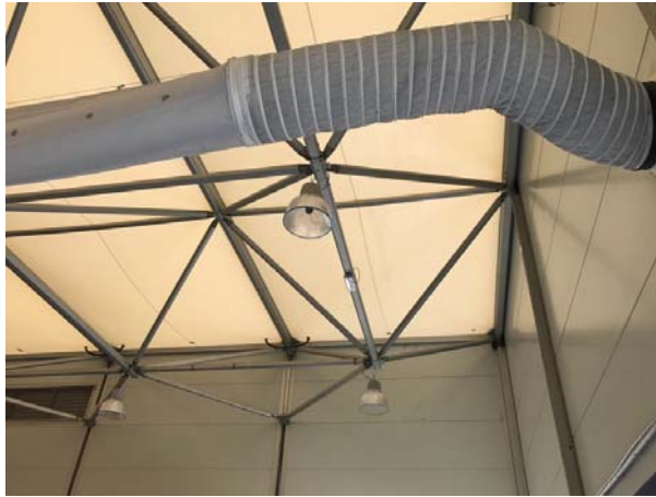
Internal Tubing for Heating and Cooling
