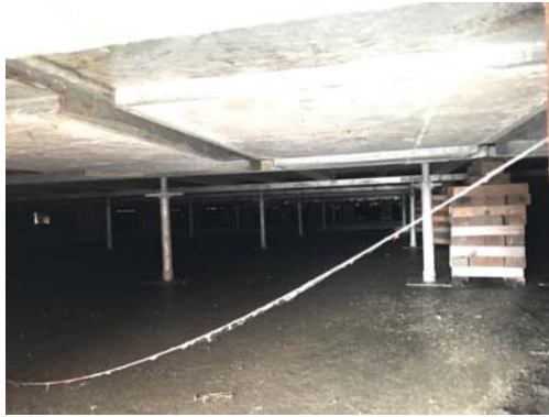
Supporting Structure Underneath Building
