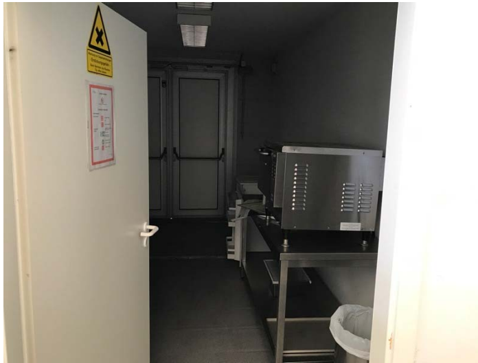
Screening Unit for Explosives Detection (Automated Trace- Explosives Detection)
