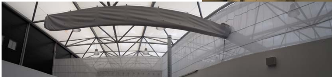
Internal Tubing for Heating and Cooling
