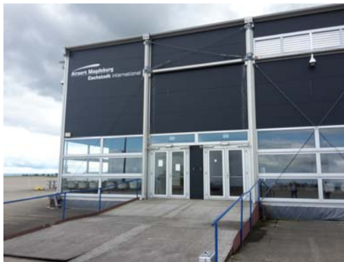
Gate 2 - Ramp Access (right door unit)
