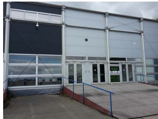
Gate 2 - Ramp Access (left door unit)
