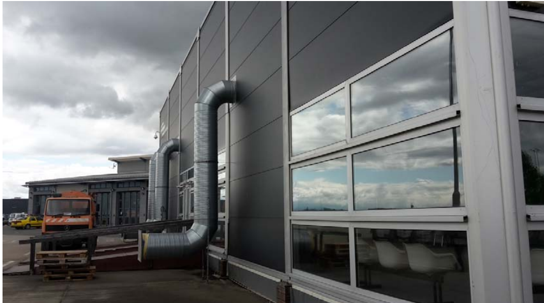
Outside Connectors for Heating and Cooling Units
